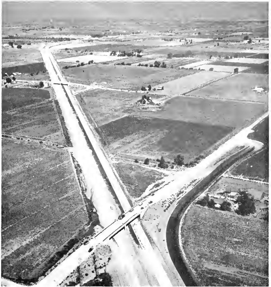
Aerial view of Manteca Freeway, looking south, showing Cottage Avenue and Louise Avenue separation structures
